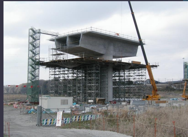
CIP upper structures
