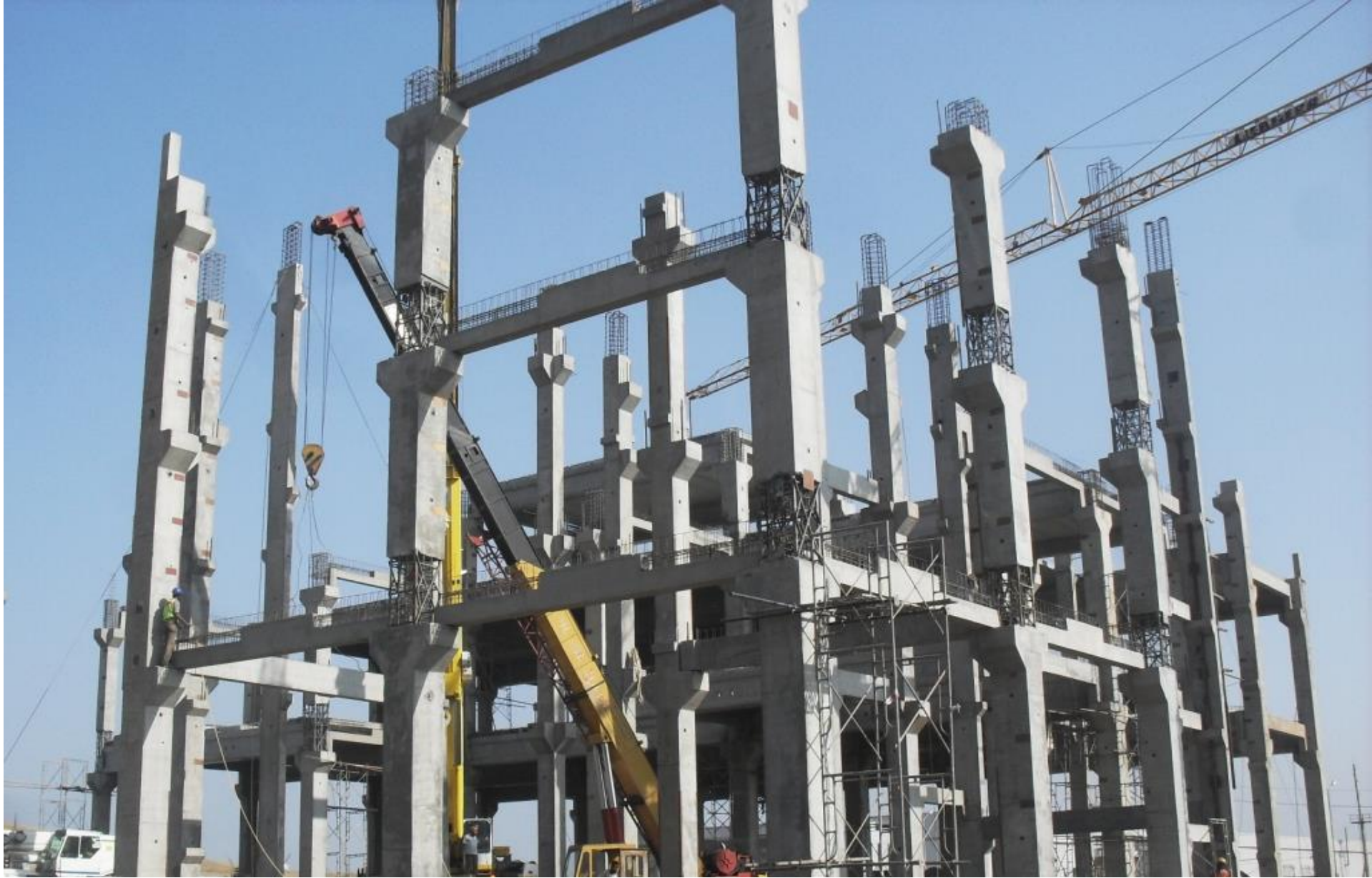
Application of Emulative System S7 (with continuous columns) in Pune-India (courtesy of Precast India Infrastructures PVT LTD - photo by Nagesh Kole)
