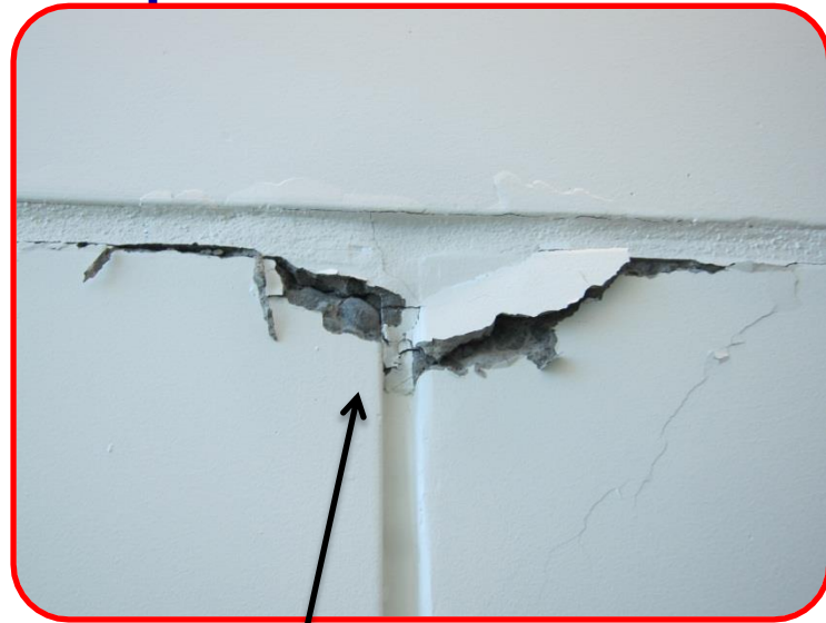
Precast walls top edges – minor crushing
