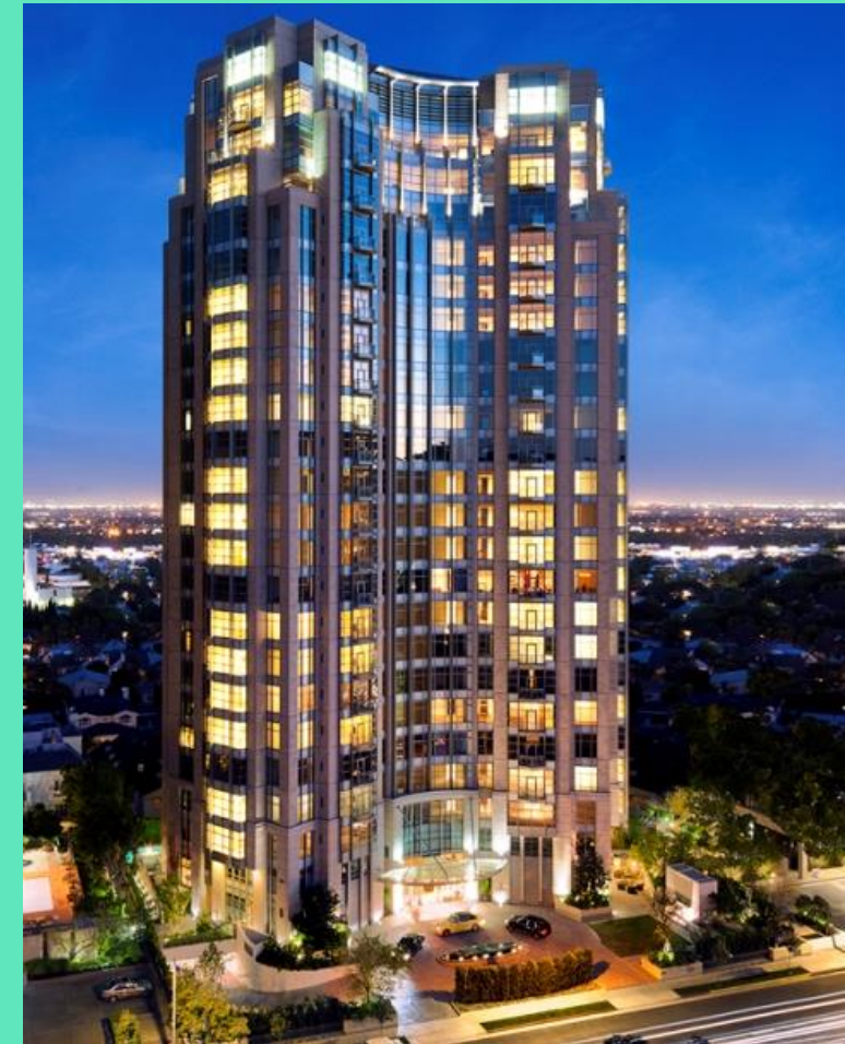
External cladding covering the structural frame at The Carlyle, Los Angeles, USA
