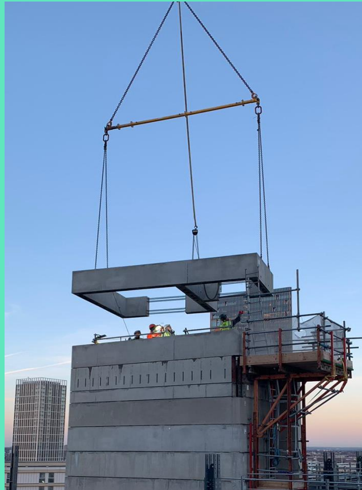
Double shaft segments with horizontal jointing only
