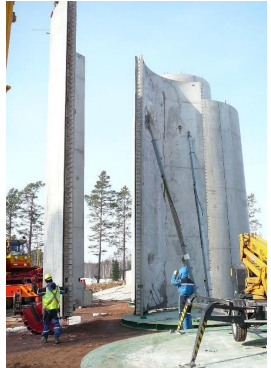
Concrete Wind Tower Assembly in Brasil (Calter)
