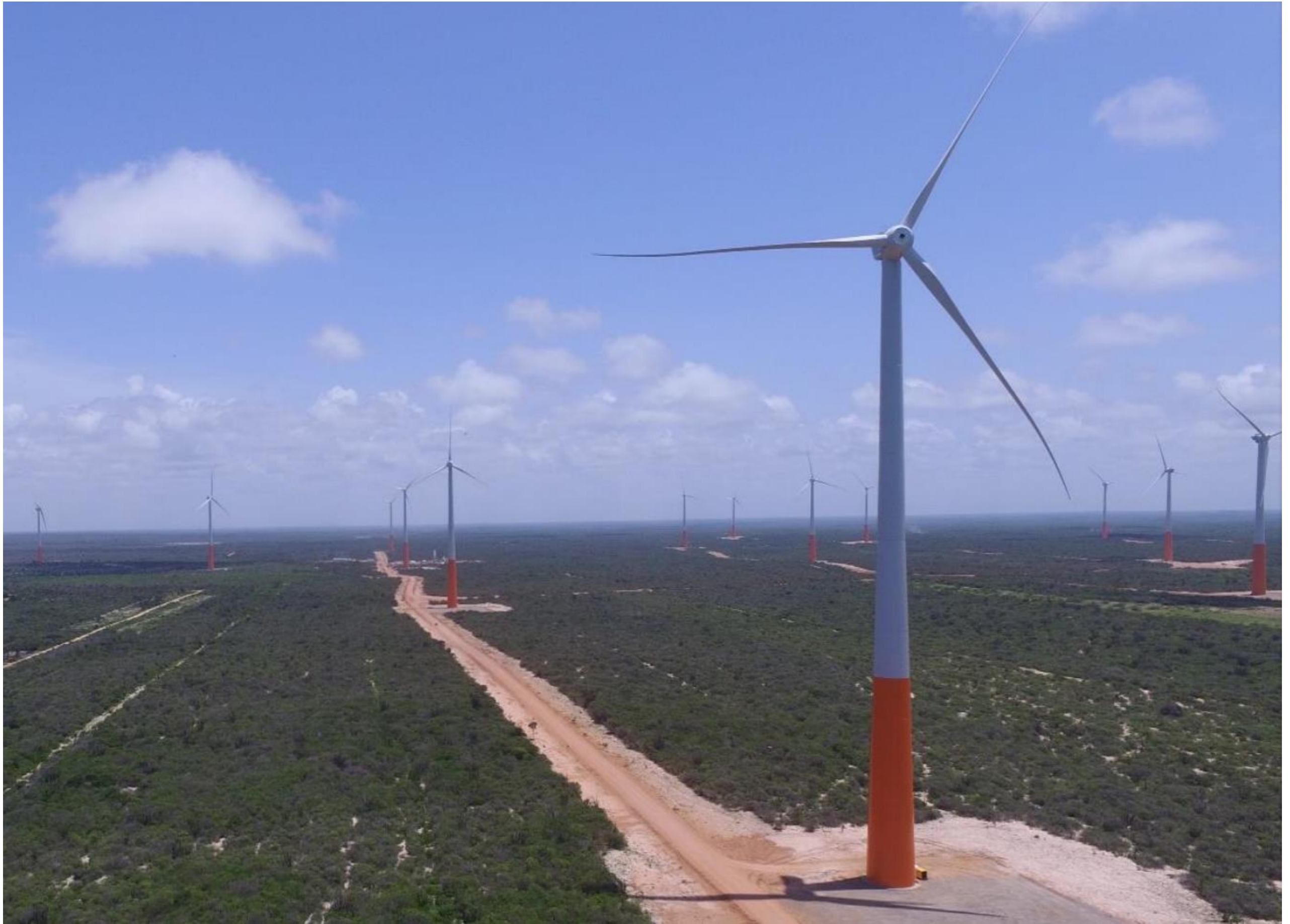
47 Concrete Wind Towers farm in production in Brasil (Calter)
