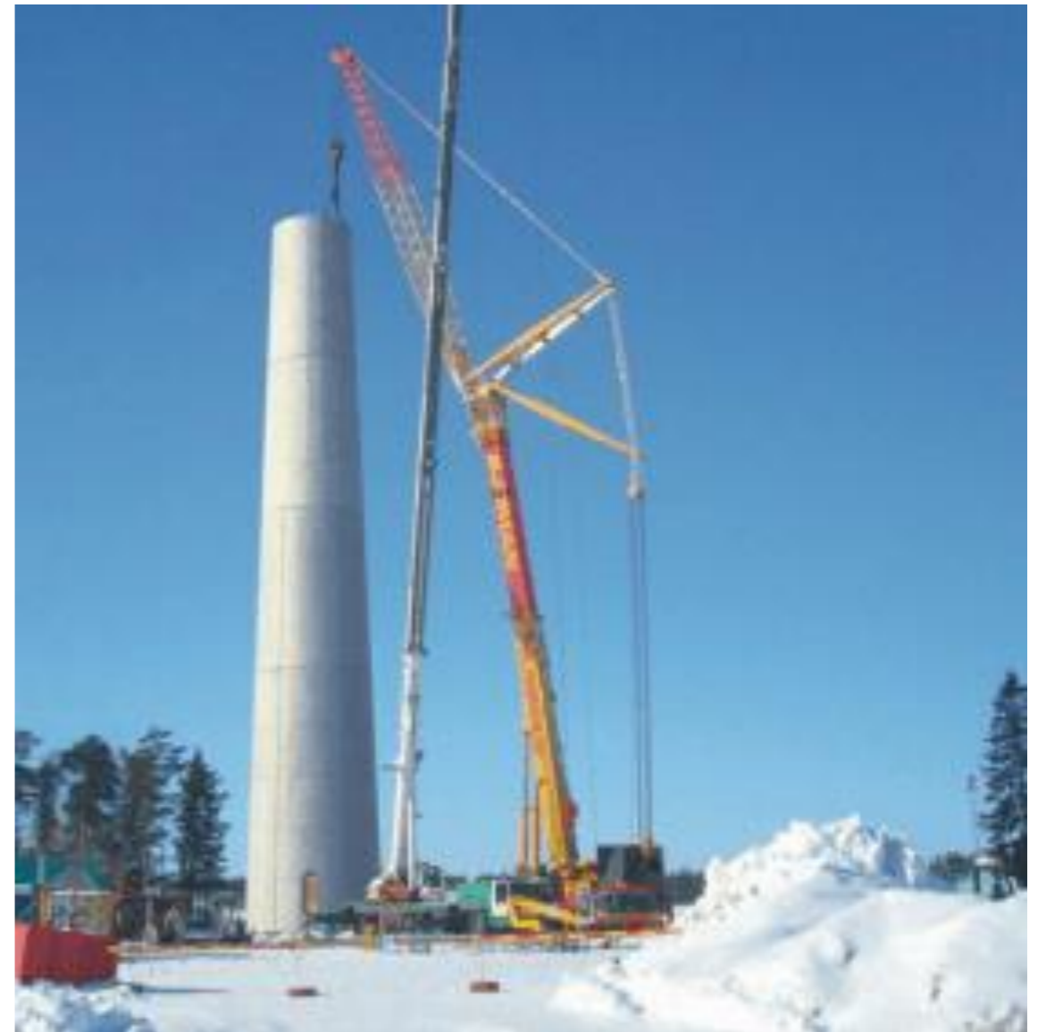
Concrete Wind Tower Assembly in Finland (Calter)
