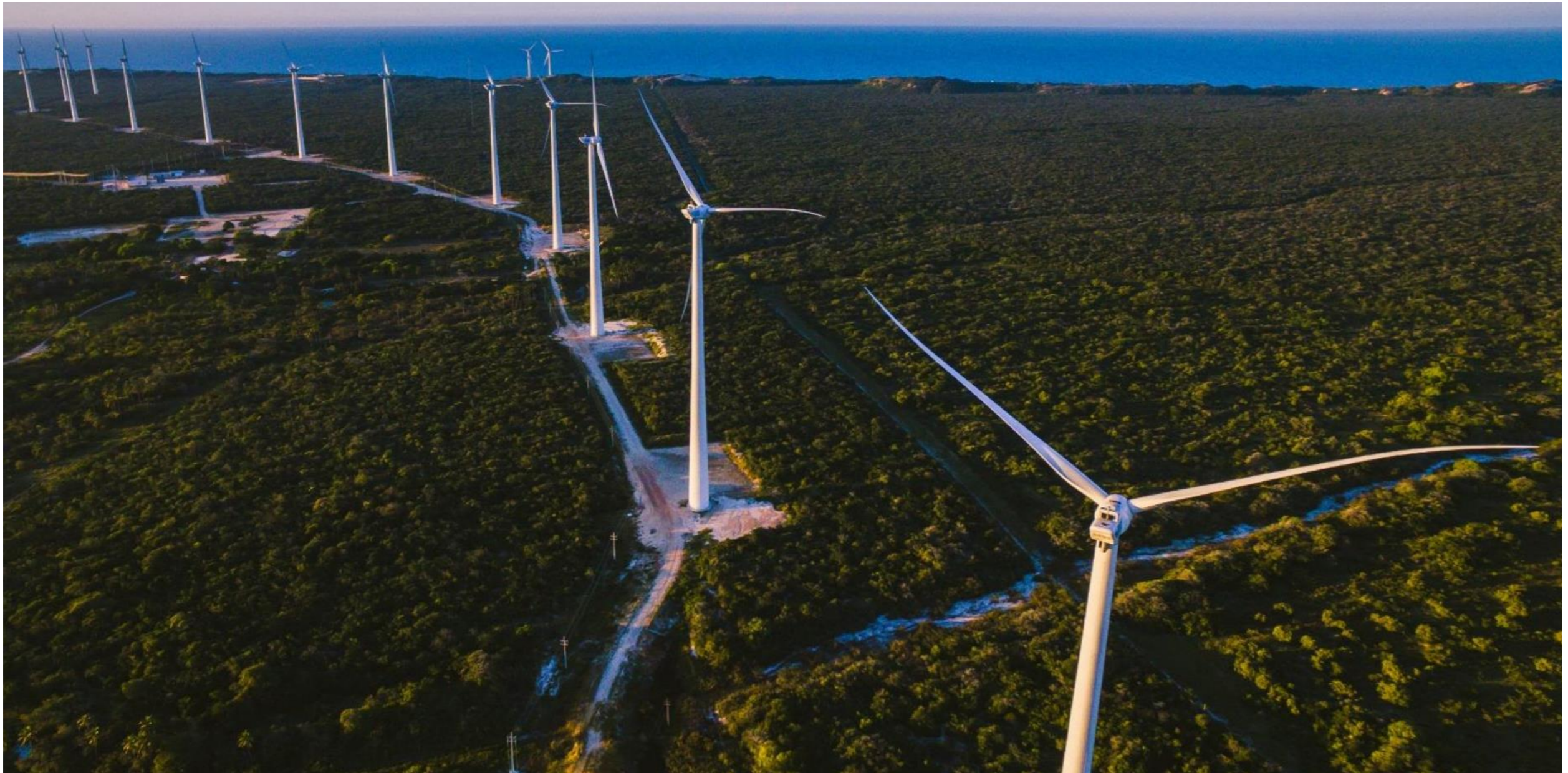
46 Concrete Wind Towers farm in production in Brasil (Calter)
