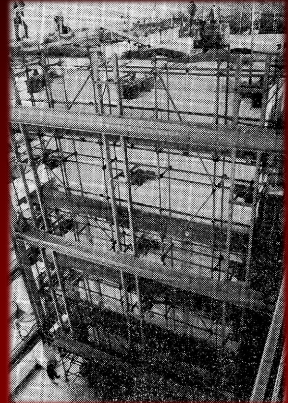
5-story precast wall building
