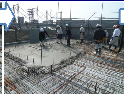
cast-in-place concrete
