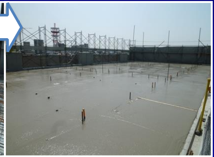
cast-in-place concrete
