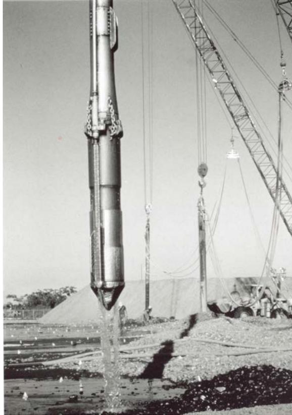
**Figure 5-4. Suspended vibrator.**
