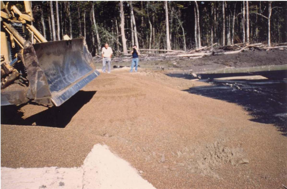
**Figure 3-5. Placing expanded clay fill.**
