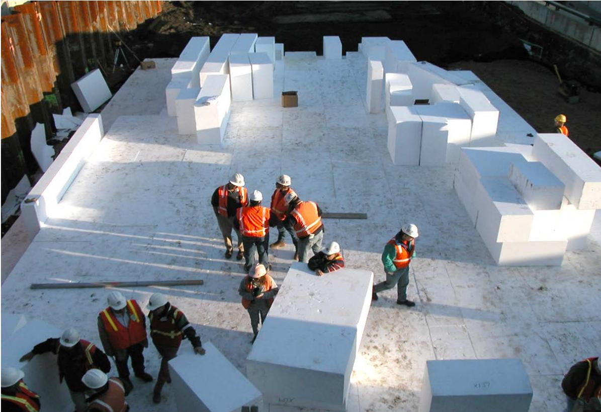
**Figure 3-1. Embankment construction with EPS-block geofoream.**
