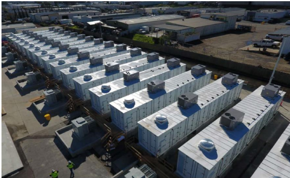
Figure 6 AES 30 MW (120 MWh) Li-Ion ESS Installation in San Diego, CA [19]
