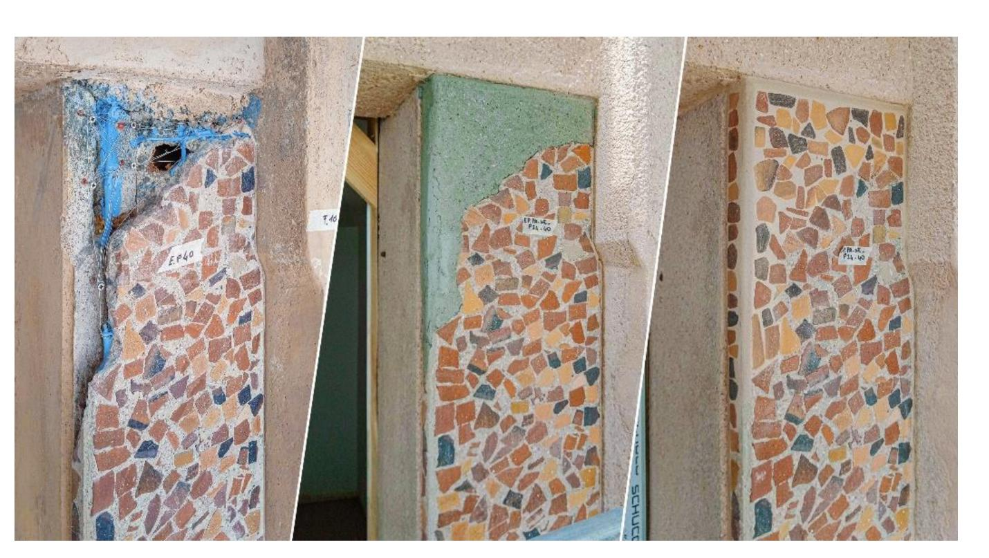
Sandblasting, manual demolition, rebars passivation, reconstruction, pictorial integration, water-repellent treatment
