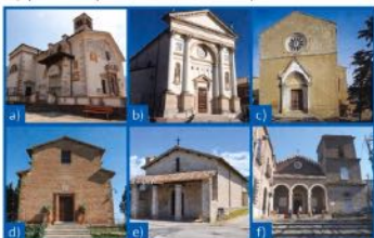
72 URM Italian medieval churches. (Pirchio et al., Construction and Building Materials, 2022)
