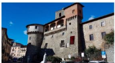
Rocca Ariostesca di Castelnovo Garfagnana (Toscana). (Oriando, Becattini, Betti, Journal of Building Engineering , 2023)
