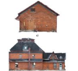
Masonry house in Kemptville, Ontario, Canada. (Farcaslu & Putasu, 2025)
