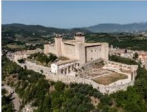
Rocca di Spoleto (PG). (Castori et al., Bulletin of Earthquake Engineering , 2018)
