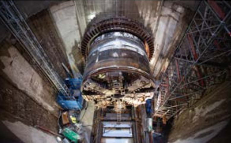
Foto 2. Breakthrough Pozzo 5.4 (© Metro C scpa)
